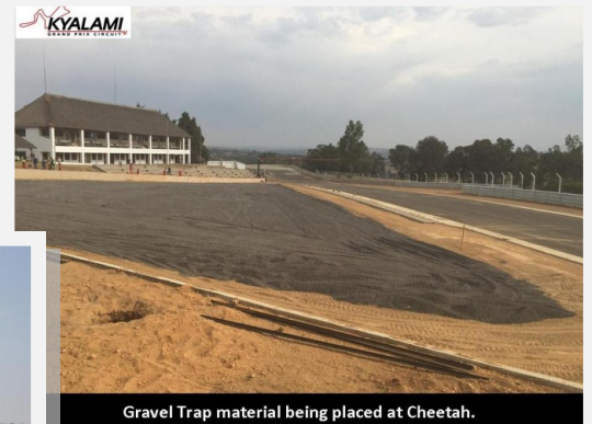
Gravel Trap material being placed at Cheetah.
