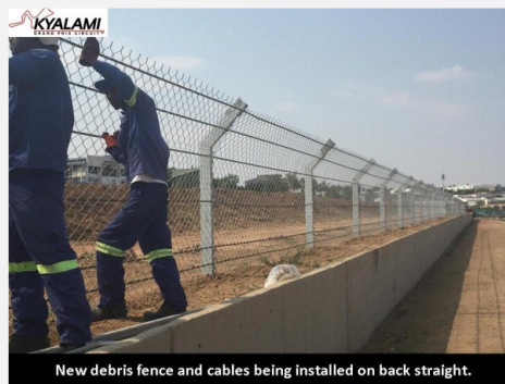
New debris fence and cables being installed on back straight.
