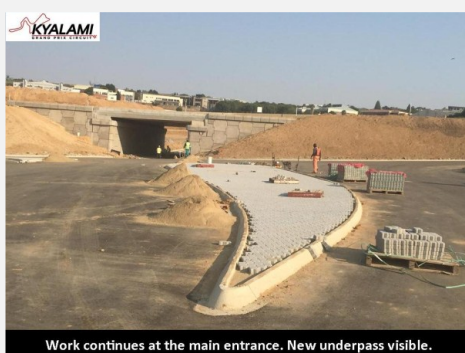
Work continues at the main entrance. New underpass visible.
