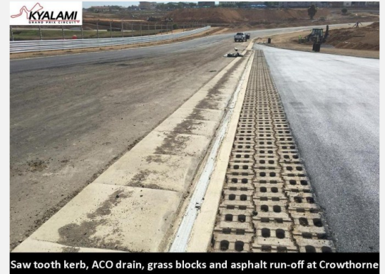
Saw tooth kerb, ACO drain, grass blocks and asphalt run-off at Crowthorne
