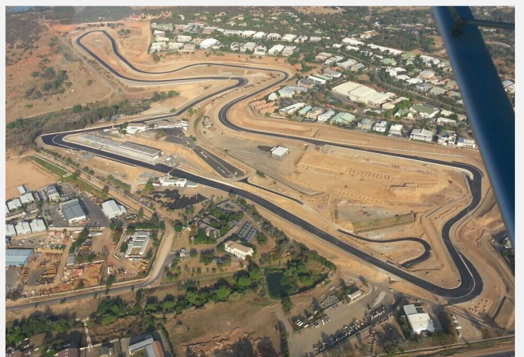
Willie du Toit (WSP) overseeing the commencement of the start of the final asphalt layer application on the back straight.
