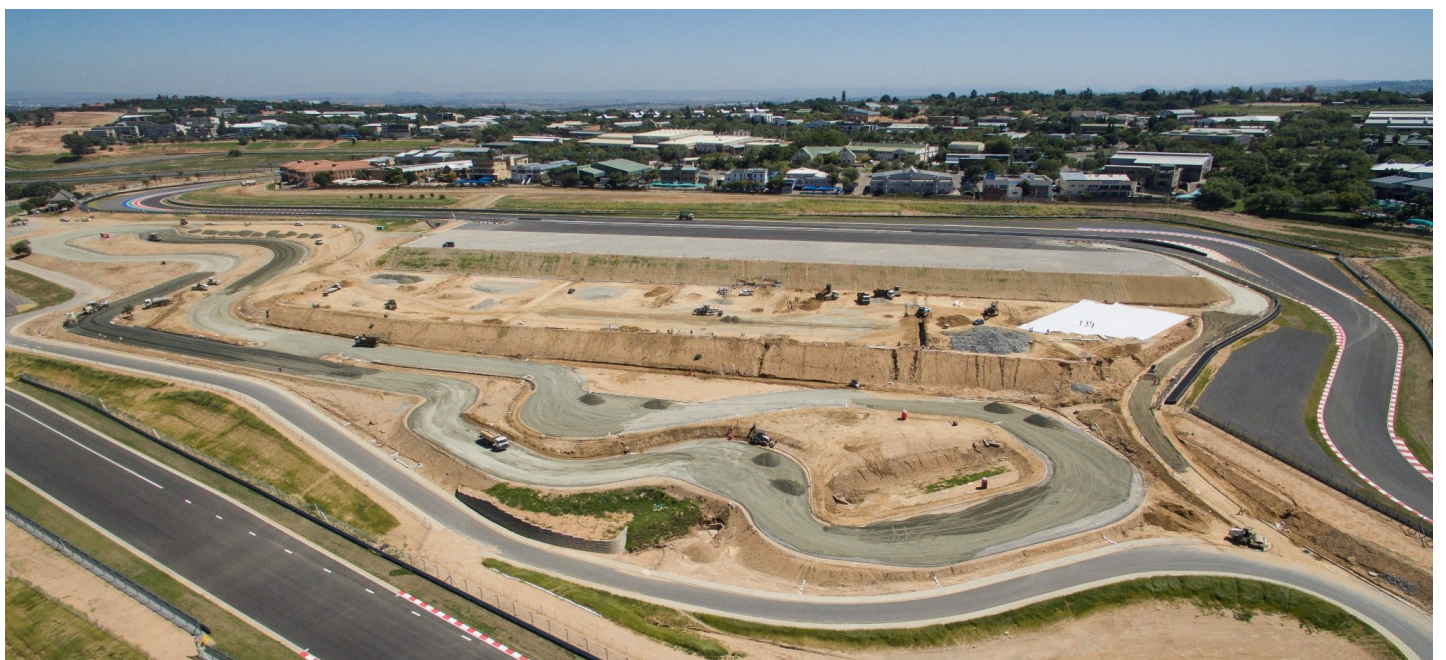
The lower section of the 1.1km handling circuit being prepared for asphalt surface. The lower platform and skidpan area is still under construction with the upper platform, now complete, visible above.
