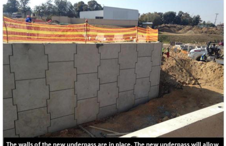
The walls of the new underpass are in place. The new underpass will allow for 2 way road traffic (transporter height) plus 2 pedestrian lanes.
