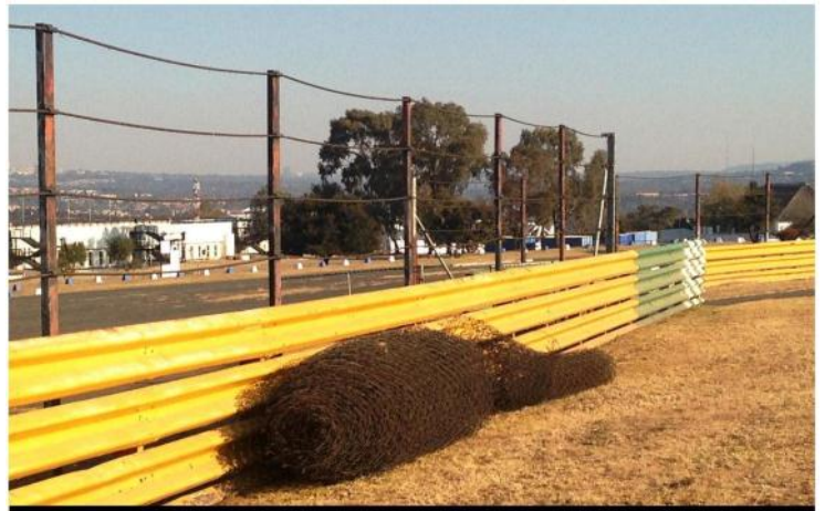
Debris fencing around the circuit is being replaced to conform to the latest FIA requirements. Over 50 km of cable is currently being manufactured.
