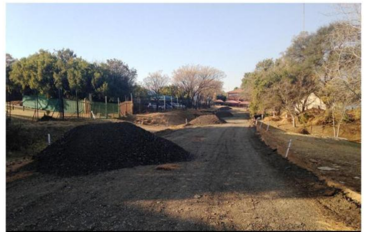
The service road around the back of the circuit will be tarred using the top layers of tar removed from the actual circuit.
