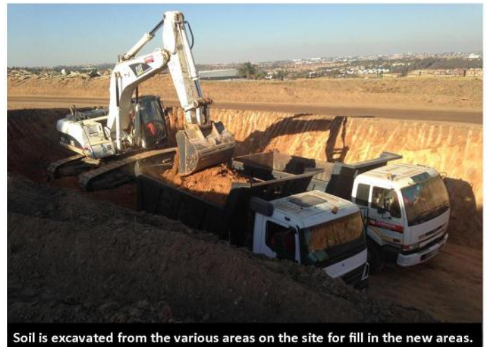
Soil is excavated from the various areas on the site for fill in the new areas.
