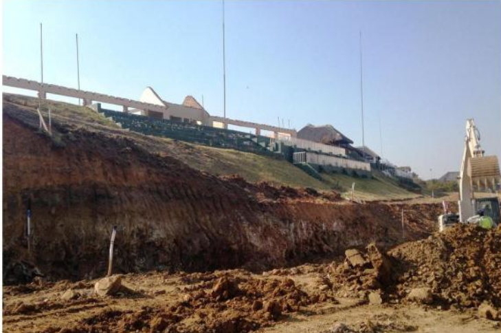
Excavations on the retaining wall at The Crocodiles, stripped bomas above.
