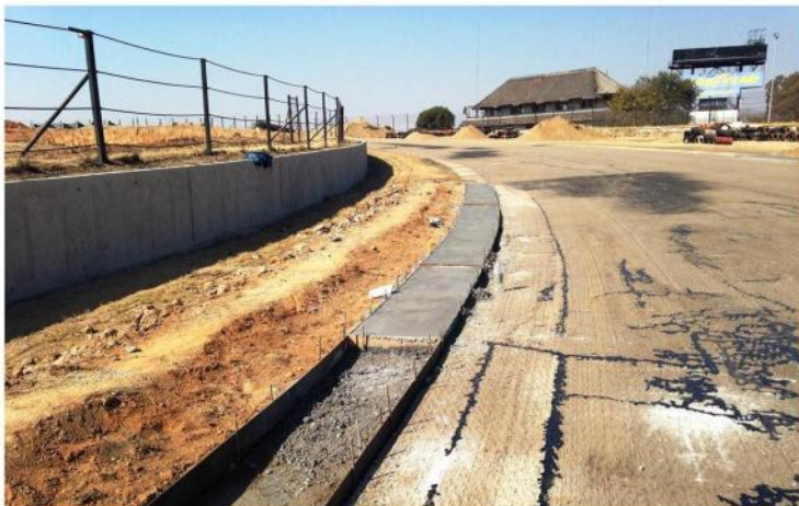
Replacement of kerbs at Sunset corner, paint stripped from the walls and fencing removed. Debris fence poles and cables still to be removed.
