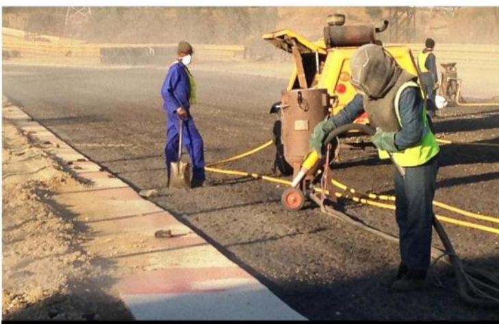
Stripping of all old paint from the concrete retaining walls and kerbs continues. Speculation on the new curb colours for the circuit continues.
