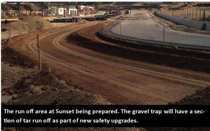
The run off area at Sunset being prepared. The gravel trap will have a section of tar run off as part of new safety upgrades.
