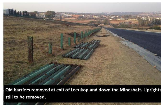
Old barriers removed at exit of Leeukop and down the Mineshaft. Uprights still to be removed.
