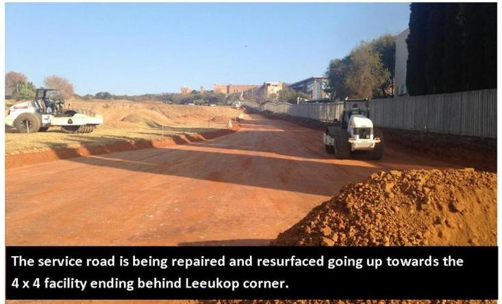
The service road is being repaired and resurfaced going up towards the 4 x 4 facility ending behind Leeukop corner.
