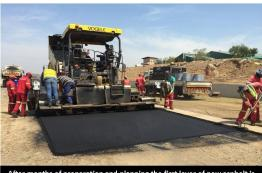
After months of preparation and planning the first layer of new asphalt is laid onto the track. A historic moment and landmark day in the proje
